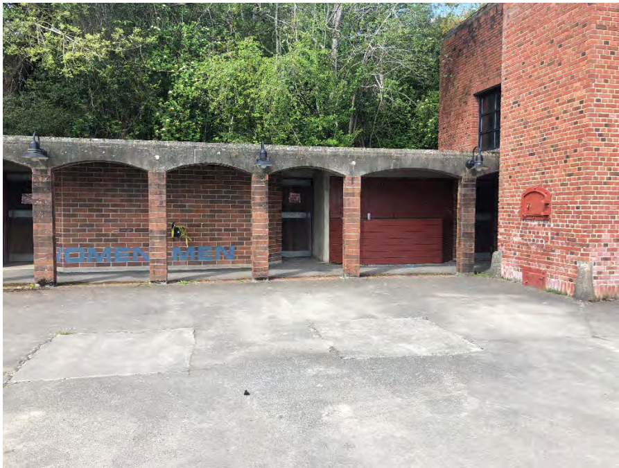
Photograph 6. Existing restroom annex building (April 2021).
