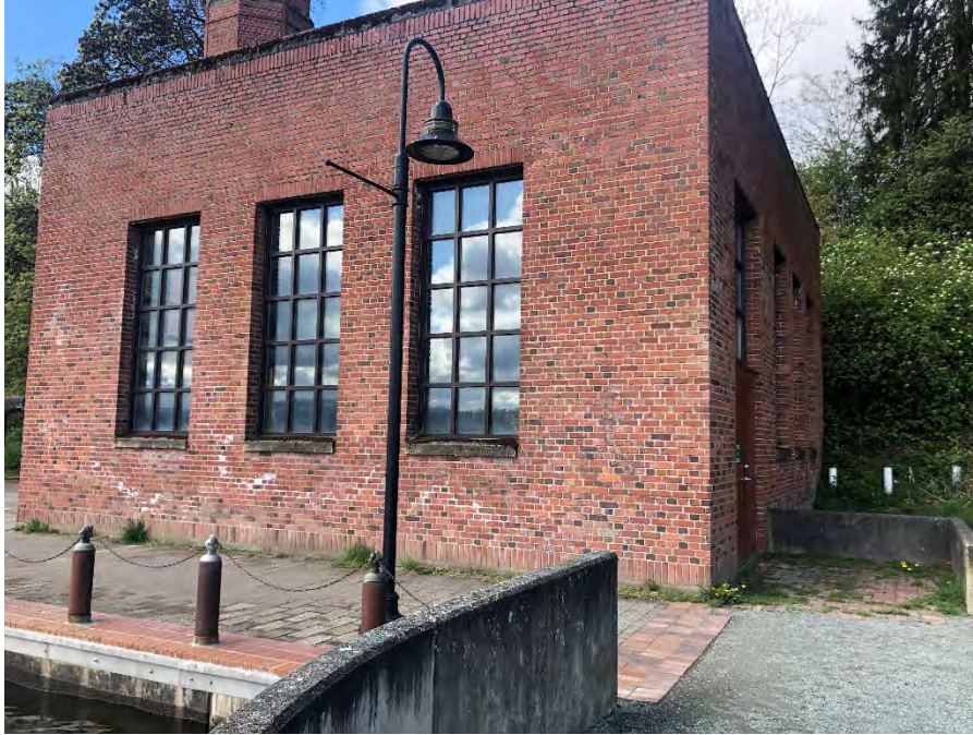
Photograph 5. Existing Boiler Building (April 2021).
